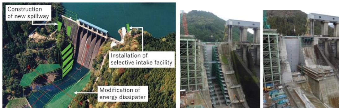
Figure 5-15 Example of intake and discharge facilities modification at Nagayasuguchi dam (Sasaki and Kondo, 2018)
