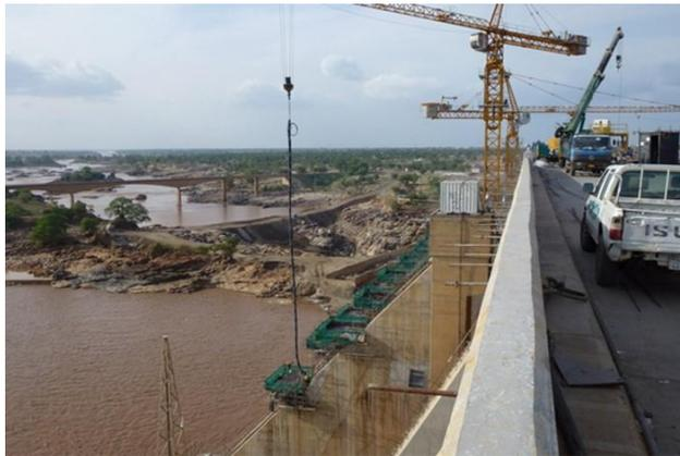
Figure 5-20 Heightening of Roseires dam (<http://pf.bbbrnetwork.com/>)
