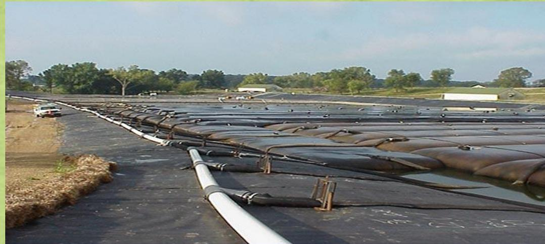
Dredged Material Cement Pug Mill / Geotube Operations (large footprint)
